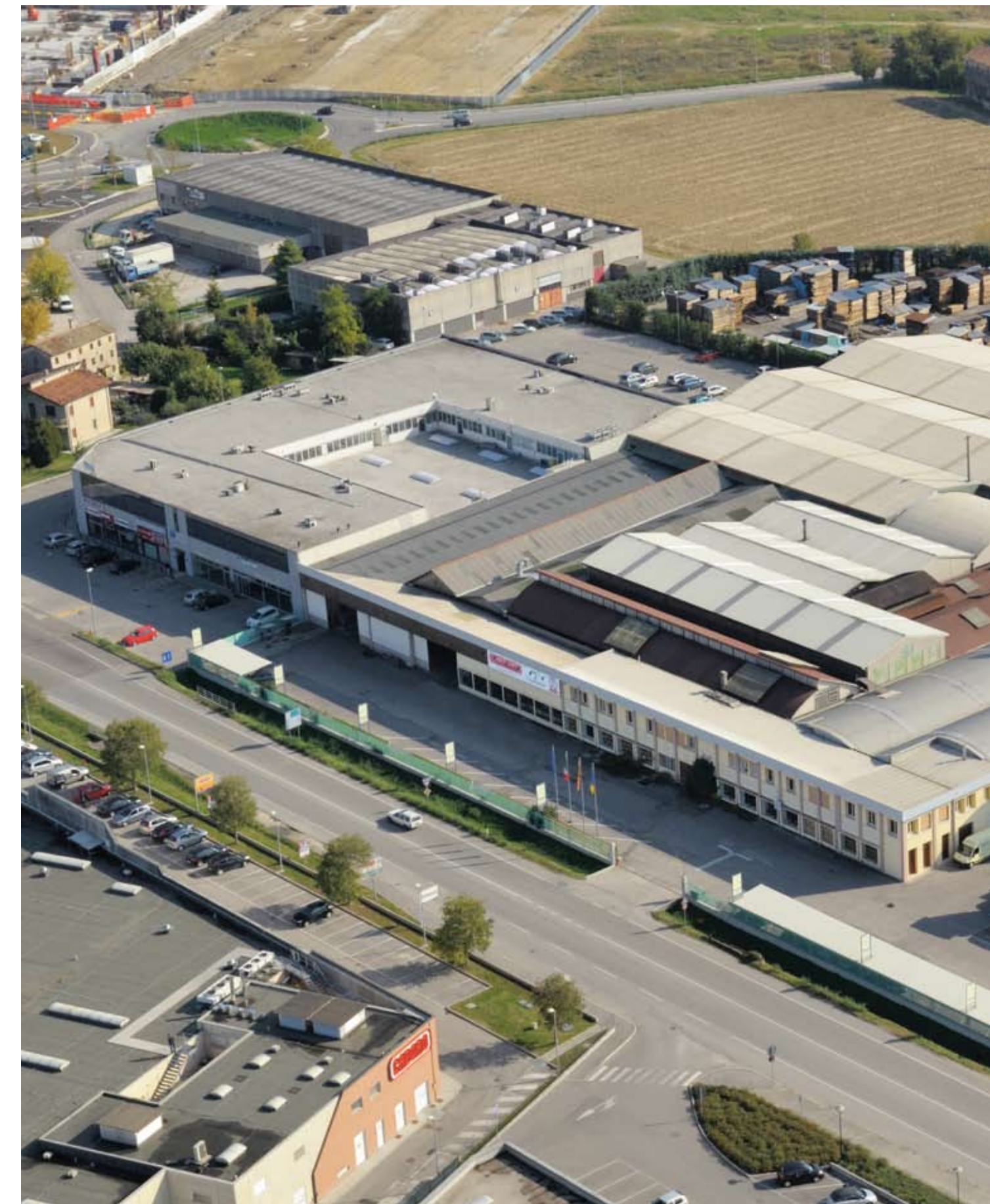
Aerial view of the industry spreading over 60,340 m 2 , 14,127 of which indoors. 15.000 m 3 of naturally seasoned wood.
