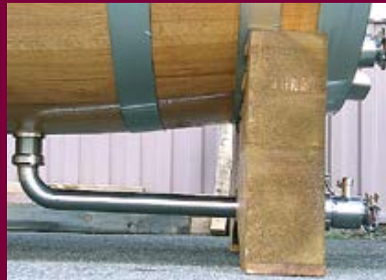
Total drainage pipe in stainless steel 18/8 AISI 304 Complete with final valve as requested, fitted to one centralstave at the bottom of the cask.
